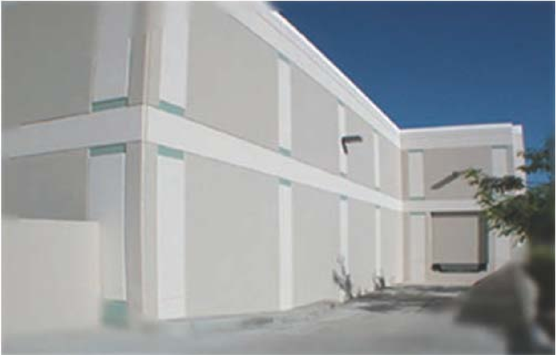
Commercial Repainting of Exterior Building
